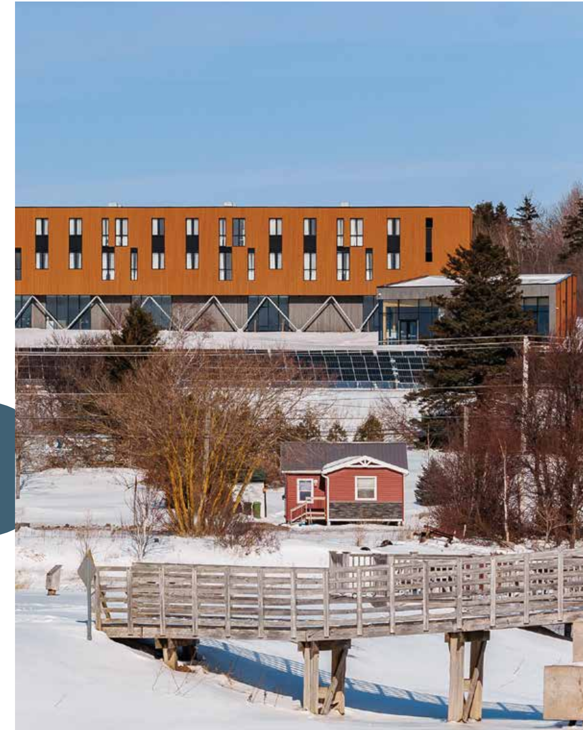
Canadian Centre for Climate Change and Adaptation (St. Peter's Bay, Prince Edward Island) by Baird Sampson Neuert Architects (now a part of WF Group Inc.) in association with SableARC Studio;
